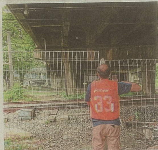
RAC worker installing a new fence along the railway tracks at Jalan Gedung Raja Abdullah in Klang.
