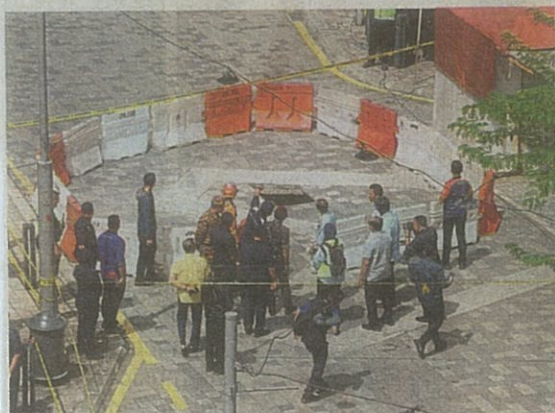
Second sinkhole about 50m from the first incident in Masjid India which cost the life of a tourist.
