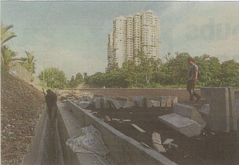
Parking facilities and drainage upgrades are being carried out at Panorama @ Bukit Antarabangsa.
