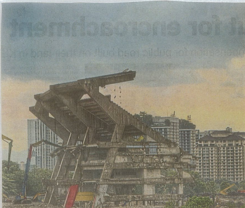
The process of demolishing Shah Alam Stadium began in stages this year. The new Shah Alam Sports Complex is projected to be completed by 2027.
