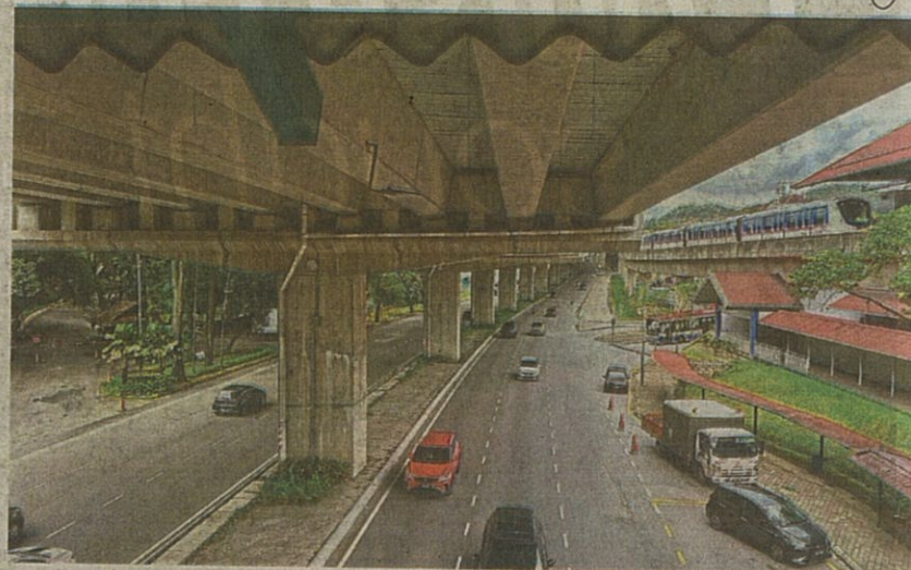
Kampung Warisan Condominium (left) is situated near Setiawangsa-Pantai Expressway (above, centre) and Setiawangsa LRT Station. — Photos: SHAARI CHEMAT and LOW BOON TAT
