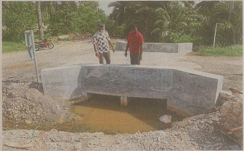
(From left) Murugan and another resident, V. Ganesan, standing on the bridge in Kampung Ampar Tenang that replaces the temporary one which the villagers had helped to build. — Photos: ART CHEN/The Star
