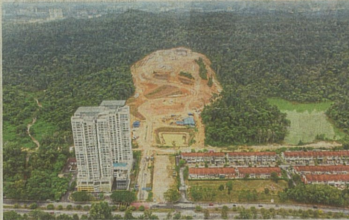
Aerial view of ongoing construction of a water treatment plant and pipeline under the Langat 2 Project. — Filepic
