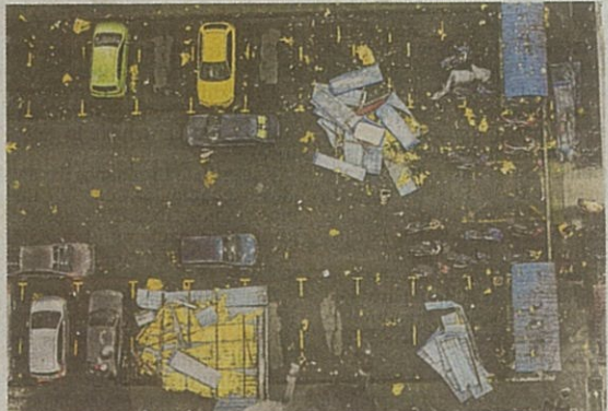
Parts of the roof scattered across a parking lot after a storm at Blok 94 of Apartment Putra Ria Bangsar on Saturday. BERNAMA PIC
