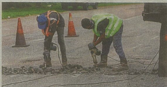
Road contractors must adopt occupational safety and health (OSH) practices at worksites. — Filepic
