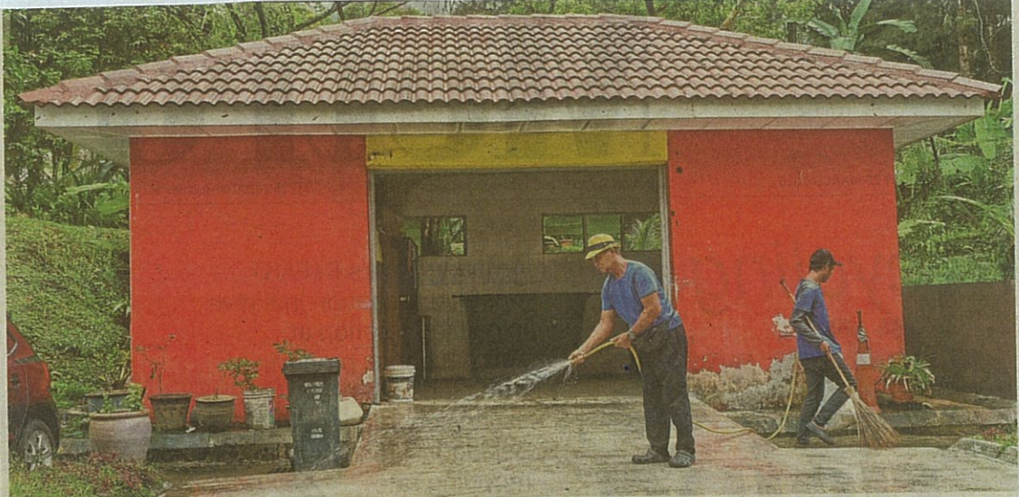
The management of Oakleaf Park Condominium utilised some of the funds generated from its waste separation project for repairs to the refuse room. — Photos: MUHAMAD SHAHRIL ROSLI/The Star
