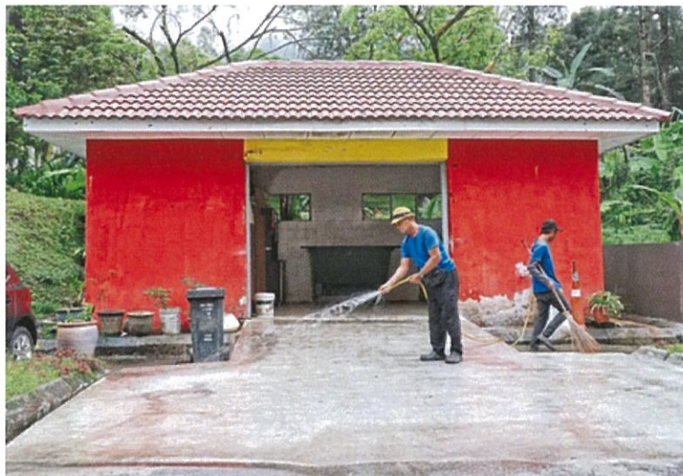
The management of Oakleaf Park Condominium utilised some of the funds generated from the waste separation project for repairs to the refuse room.
