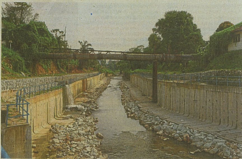
The river diversion project at Sungai Kayu Ara is among the many flood mitigation projects that have been completed in Petaling Jaya. — Filepic
