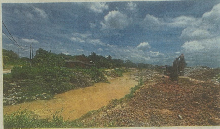
Flood mitigation works at Sungai Subang have attained only 18% completion instead of the projected 23%. — Filepic
