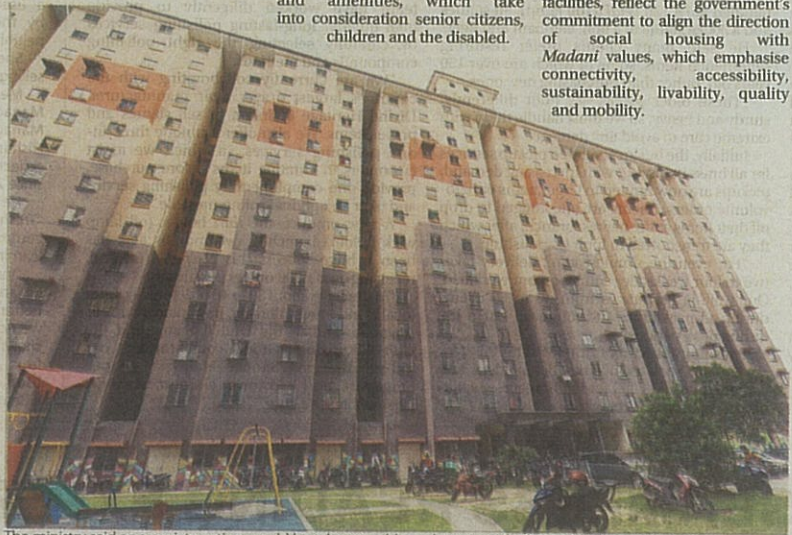
The ministry said appropriate action would be taken to address damage to facilities related to daily needs, such as water, electricity and lifts. — AMIRUL SYAFIQ/THESUN
