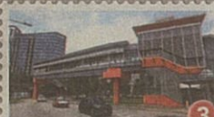
MRT Cochrane - Sunway Velocity link bridge
