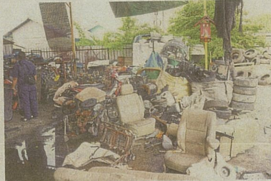
MPS demolished an illegal workshop in Kampung Melayu Sungai Buloh earlier this week.
