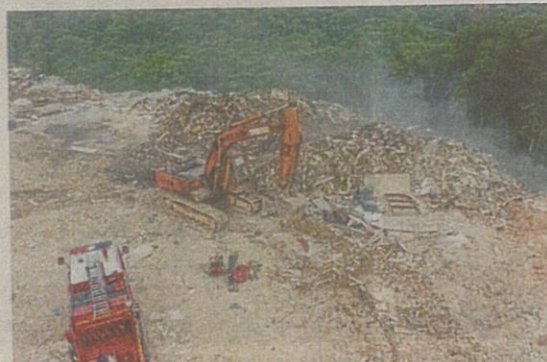
MPKj successfully rehabilitated an illegal dumpsite that had caused misery to residents for years.
