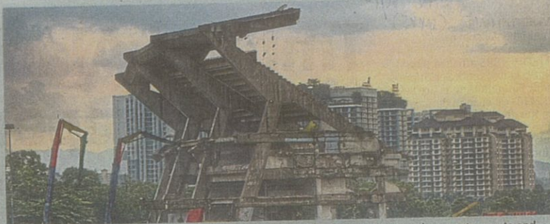
Shah Alam Stadium, which used to be the venue for football matches among other sports events and concerts, is now being demolished to make way for a new sports complex.
