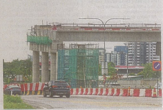
The 36km dual-carriageway EKVE has faced numerous challenges due to complex legal, financial and logistical issues.
