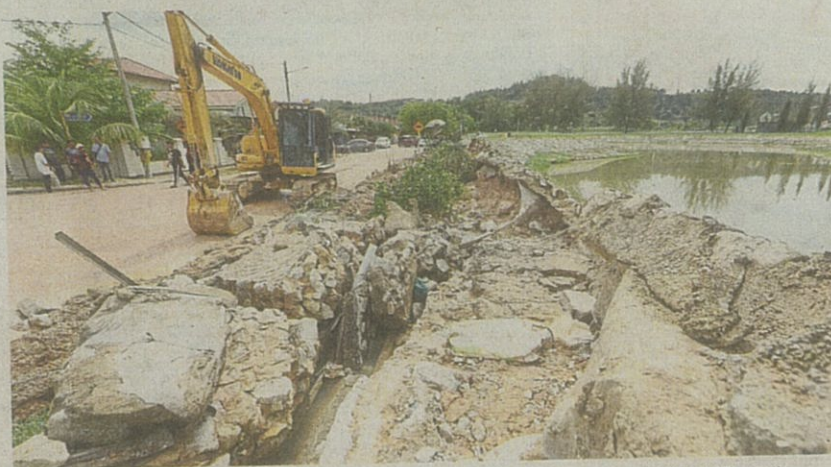
Repairs being carried out at the collapsed bund in Bandar Saujana Utama. — FAIHAN GHANI/The Star
