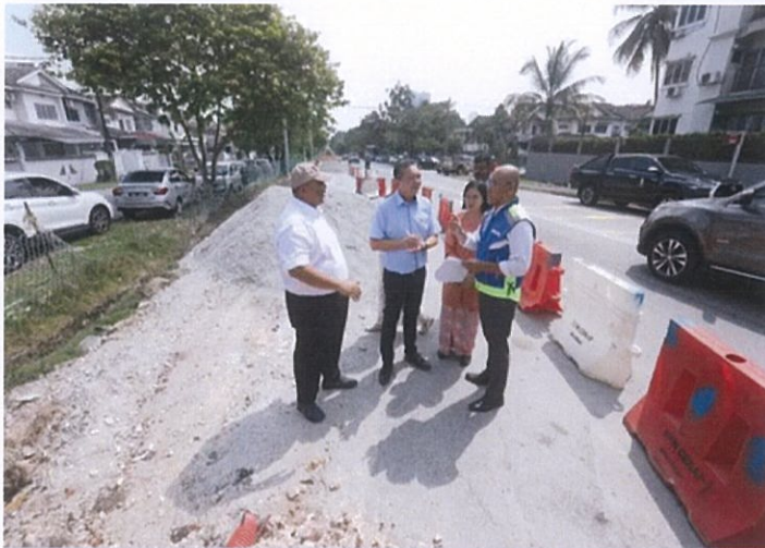
(From left) Amirul, Ng and Mohd Ariffuddin discussing the upgrade works.
