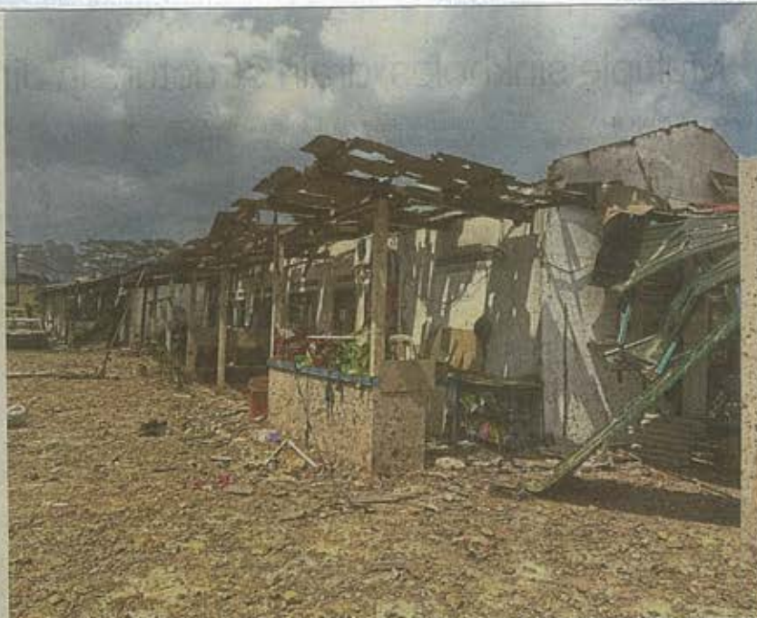
An entire row of destroyed houses in Kampung Kuala Sungai Baru which is only 400m from the gas pipeline blast site in Putra Heights. — Photos: GRACE CHEN/The Star and courtesy photos
