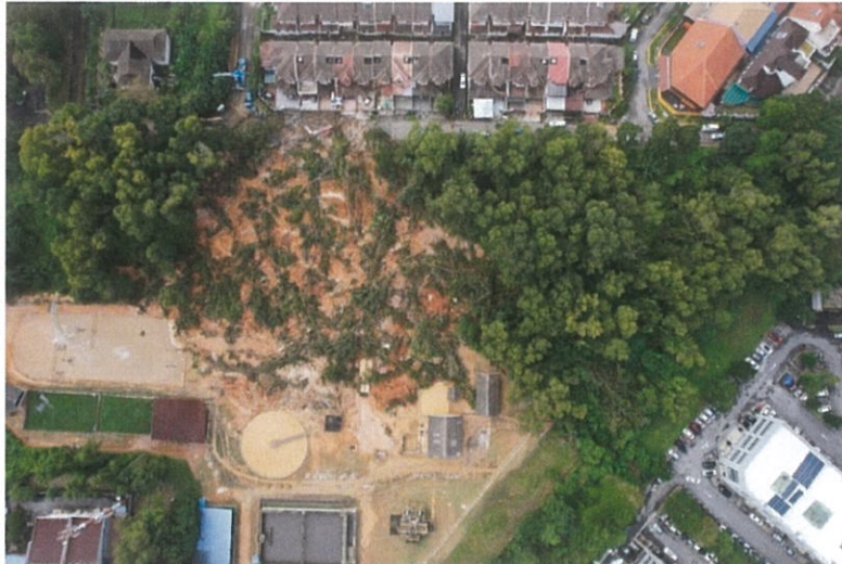
FILES: An aerial view of the landslide site in Taman Wawasan, Puchong on December 16, last year. - Filepic courtesy of Public Works Department
