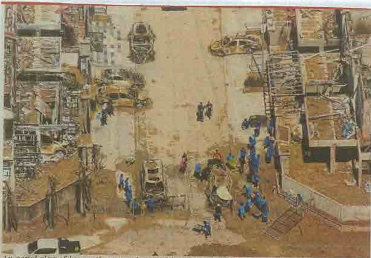
An aerial view of houses that were destroyed in the Putra Heights gas pipeline fire in Subang Jaya. SCREENGRAB FROM POLICE DRONE VIDEO
