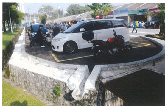
With over 1,000 visitors flocking to the trails every weekend at the Wawasan Hill in Pusat Bandar Puchong, the new parking lot is intended to deter illegal parking.
