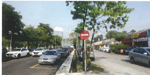
The 49 new parking lots near the Wawasan Hill Trail's at Pusat Bandar Puchong was completed Dec Last year.
