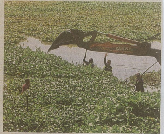
Workers seen at Sungai Midah flood retention pond in Bandar Tun Razak, Kuala Lumpur. — Photos: FAIHAN GHANI/The Star
