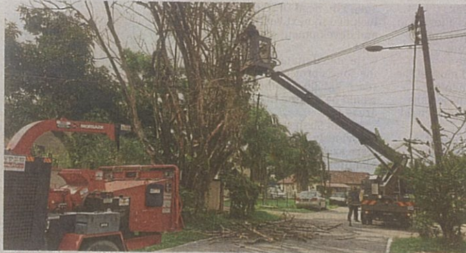
MBDK workers dealing with a dead tree at Jalan Mastika, off Jalan Mengkuang, in Klang.
