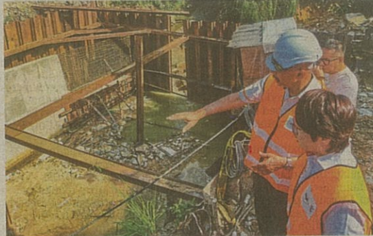
Mohamed Razeek (wearing safety helmet) briefing Pua (right) about the culvert construction during a visit to the site.
