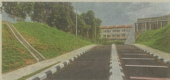
The road connecting Jalan 23/119 and Jalan 31/119 cost about RM1mil to build.
